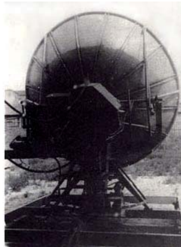
Figure 20b. The transmitter located on the back side of the radiating reflector of the Zenit antenna.
