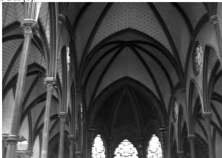
Figure 6. Louis-Auguste Boileau, Church of St. Eugène, 1854–1855, Paris, interior.
