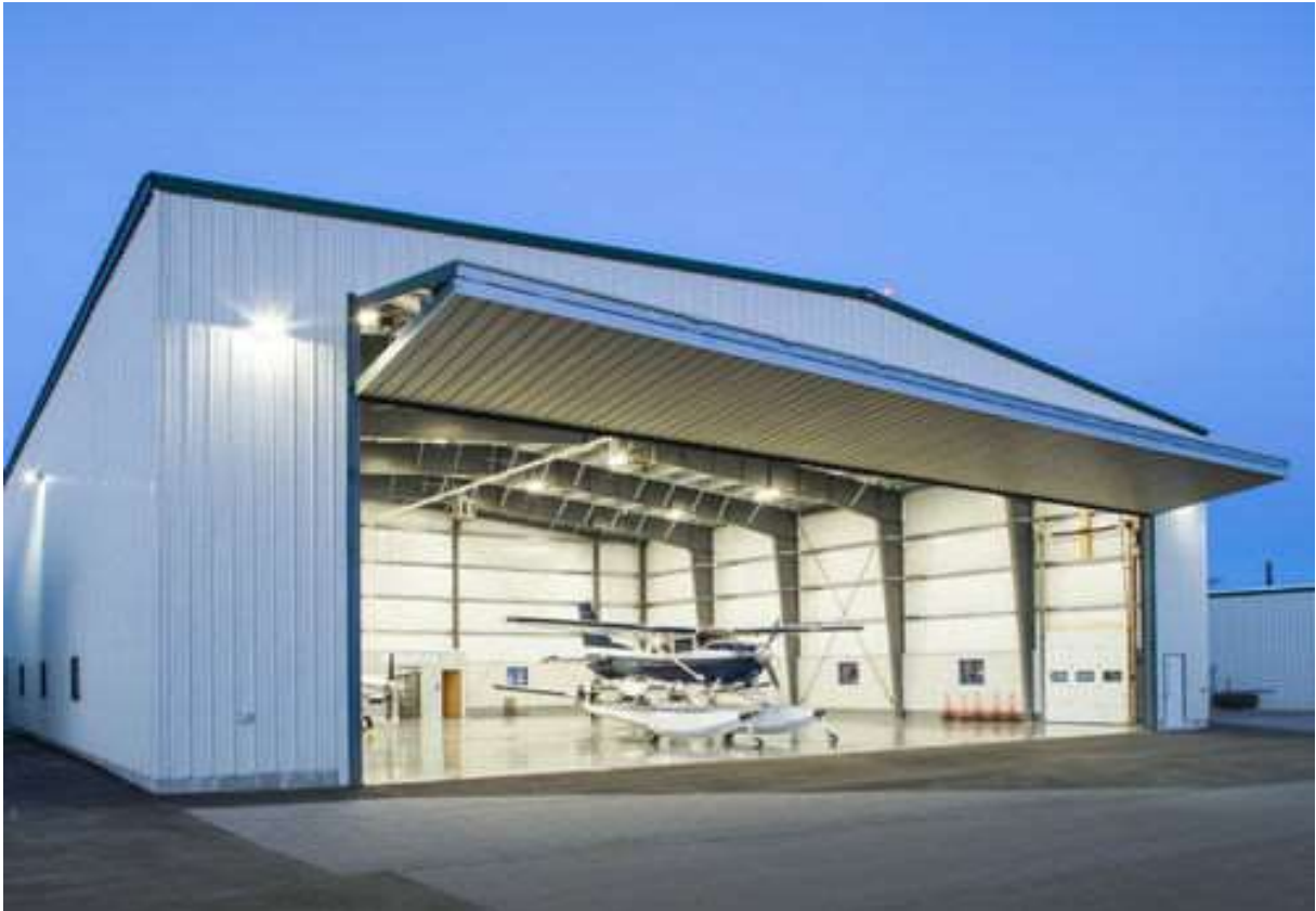
Fig.2.3.1 Staying the aircraft in the hangar for protection from snow and ice [25]
