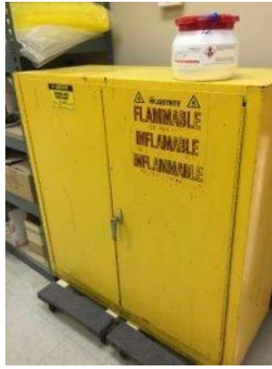
Fig. 4.3. Flammable fire cabinets.
