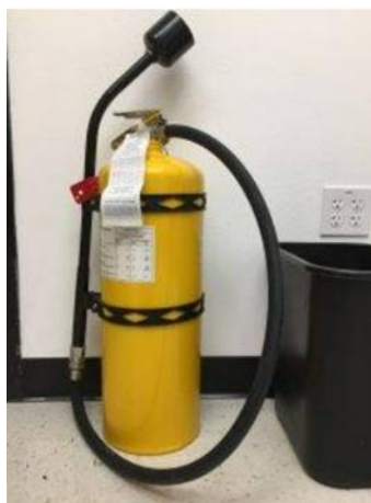
Fig. 4.2. Laboratory metal fire extinguishers.
