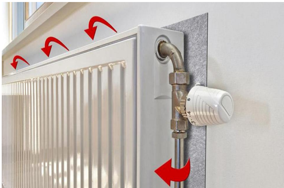
Figure 5 Heat-reflective shield behind the radiator
