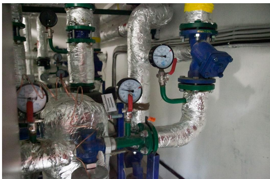
Figure 26. Individual heating point with weather control.
