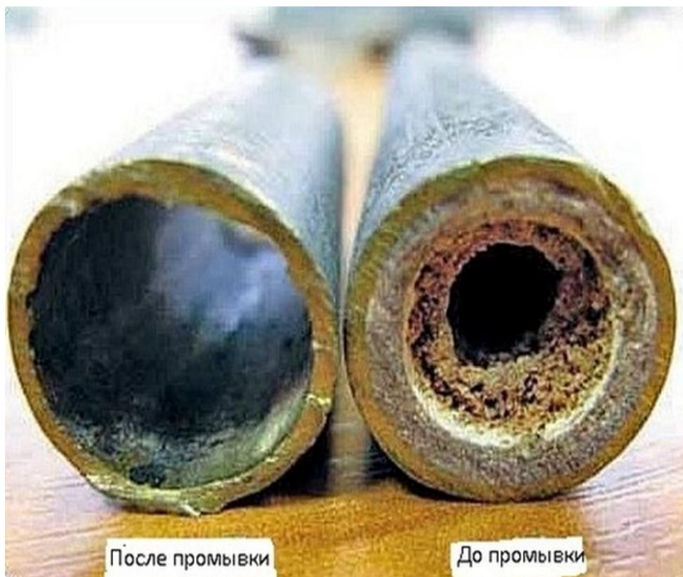
Figure 3 Comparison of the battery tube before and after flushing
