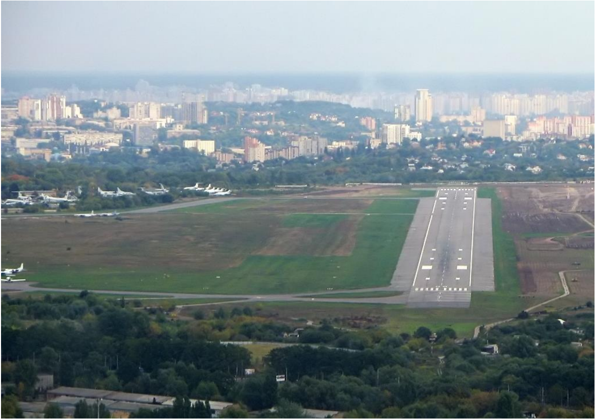
Figure 1.1 - View of the runway of the Zhulyany airfield
